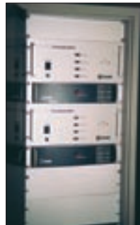
The R30 AIS Base Station and BL-10 Base Station Controller
